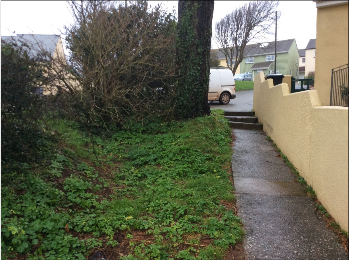
Figure 3: Point of origin from linear POS and condition of footway serving properties
