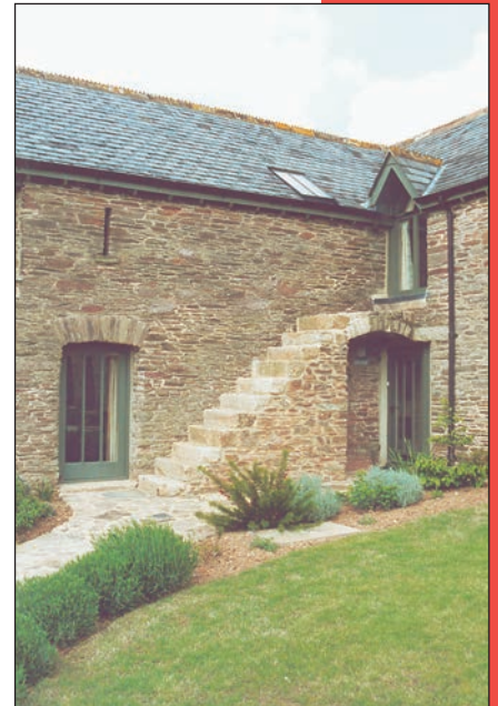
Right: Although conversion made these characterful stone steps redundant they were nevertheless retained as a feature of interest and a reminder of how the building was formerly used.
