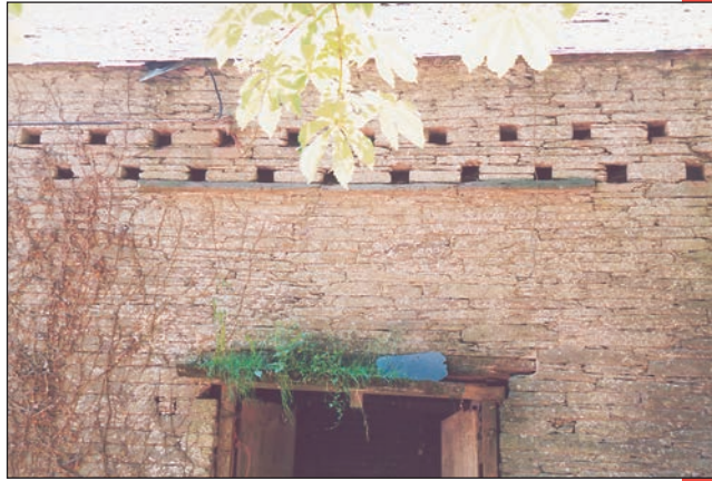
Above: The nesting holes in this 17th century farm building are somewhat unusual in that the central few on the bottom row have slate slabs running along their bases. That the slabs are above the doorway, and project out from the wall by a small and seemingly measured amount, suggests they weren't provided for the pigeons' benefit, but to spare whoever used the door from being 'spotted'.
