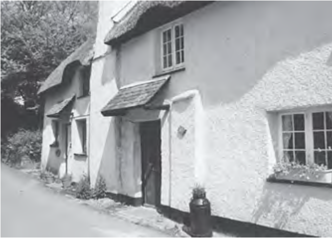
Figure 55 The 'vernacular' style of these 17th century cottages derives mainly from the informality of their appearance
